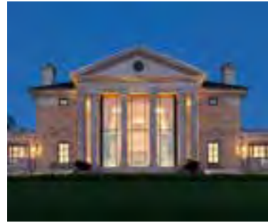
Project: V HOUSE Architect: Dalgliesh Gilpin Paxton Architects
