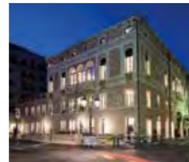
Project: PALAZZO ONIGO Architect: Geom. Barbisan - Arch. Vendrame Arch. Fioretti - Ing. Dalla Cia
